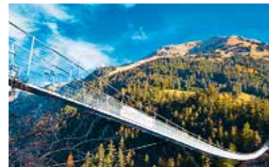
THE HOLZGAU SUSPENSION BRIDGE
